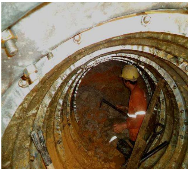
Fig. 1 - Dentro do Tunnel liner.
